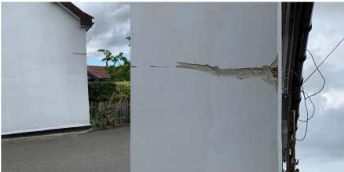
Damage to the Forge at Jubilee Corner by a passing vehicle July 2020
