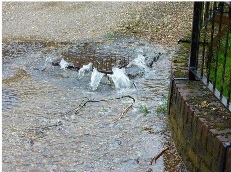
rainfall the sewer is overloaded and the manholes lift. Anglian Water confirmed that this cannot be solved as a larger sewer would result in the flows being too slow under normal conditions, resulting in odour and blockages. 24 new houses will discharge into the system thereby increasing the amount of sewage and reducing the capacity for the surface water rain. The sewage in the system will be more concentrated and therefore more polluting.
